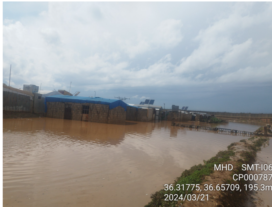
Flood Incident in Zazam2 IDp Site(Source: Muzun NGO)
