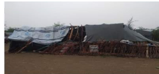
Image 3: Shelter damaged during flooding in Saylat-Alrumayla. Source: IOM
