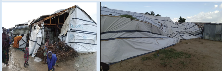
Pulka reception centre requires reconstruction with semi-permanent structure©IOM
