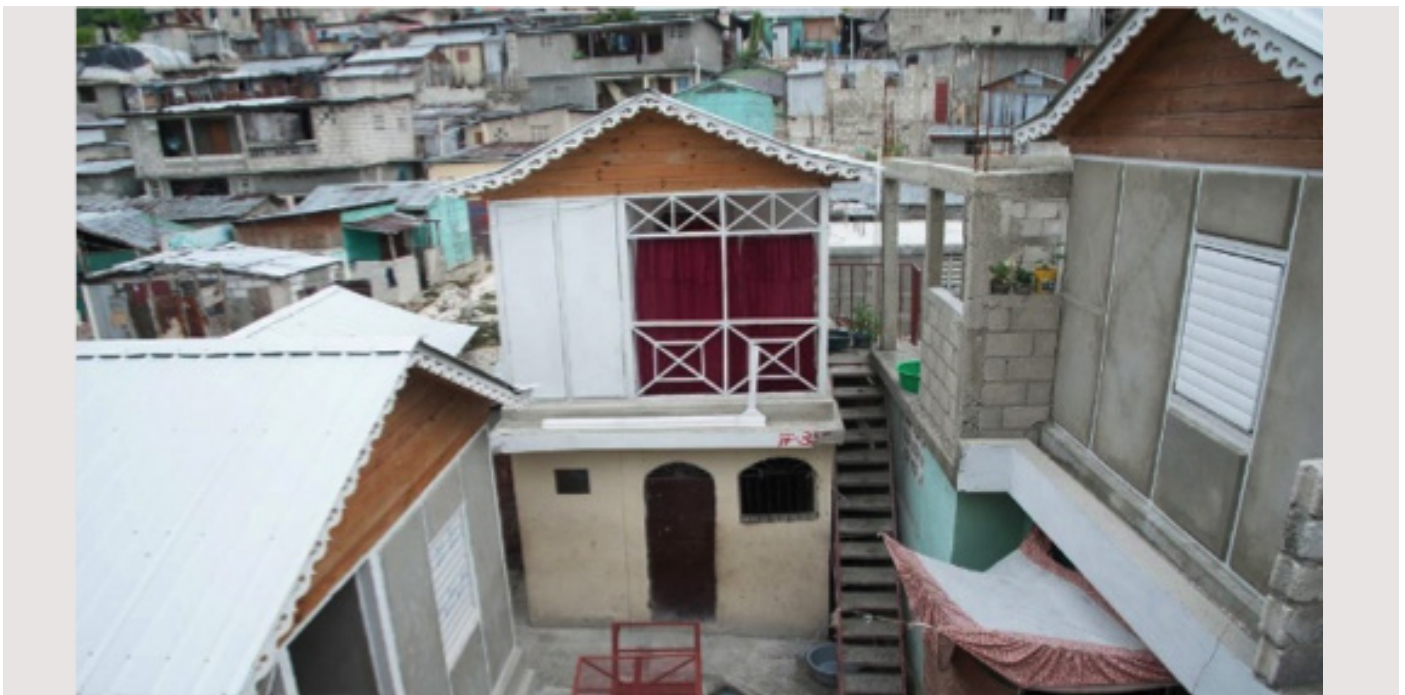
Construction and reinforcements with wooden framing
