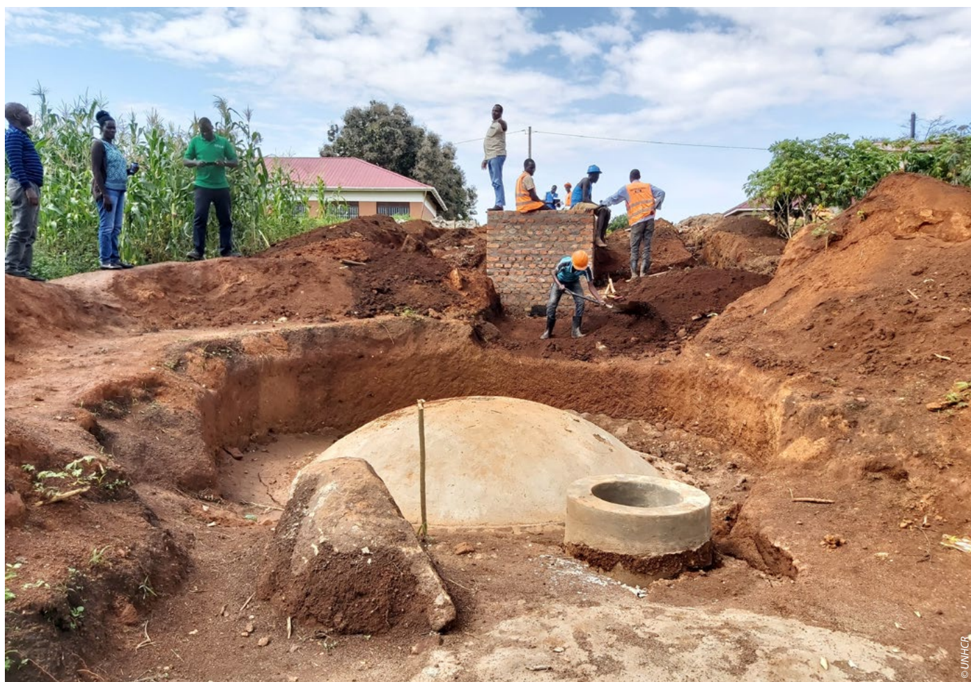
Biogas plant construction in a school in Kyangwali to reduce firewood use for cooking
